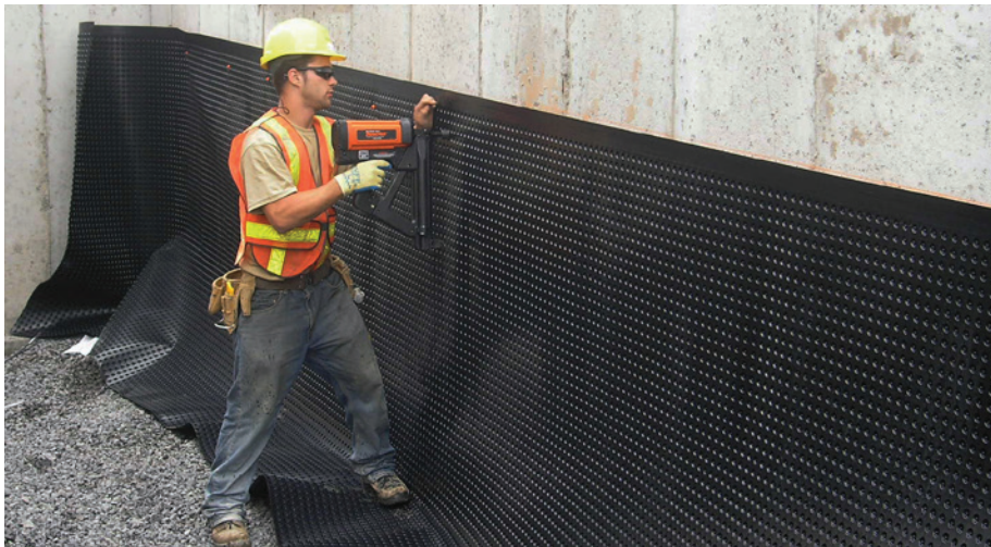
PLATON INSTALLATION - FOUNDATION WALLS
