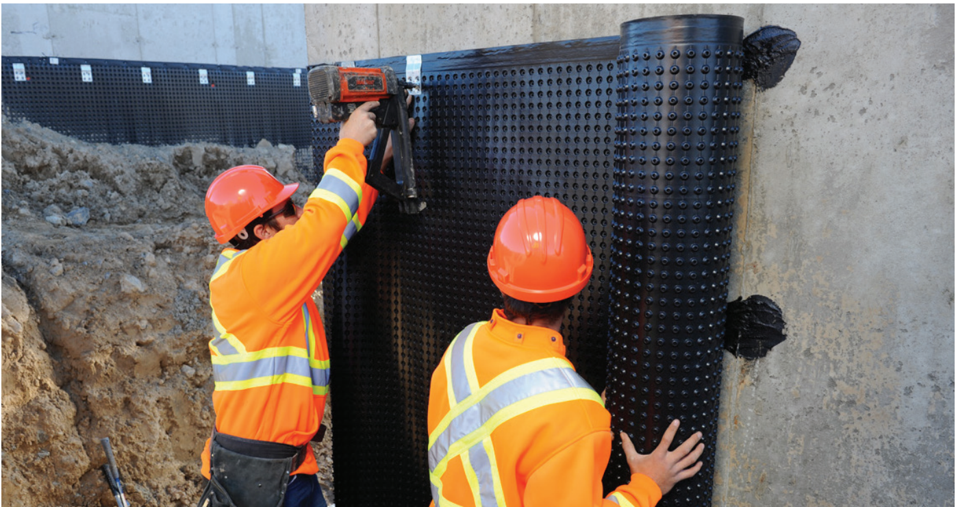
PLATON INSTALLATION - FOUNDATION WALLS
